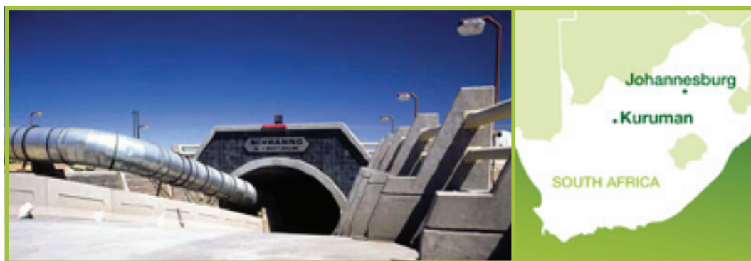
Nchwaning's 2,200 m inclined shaft
