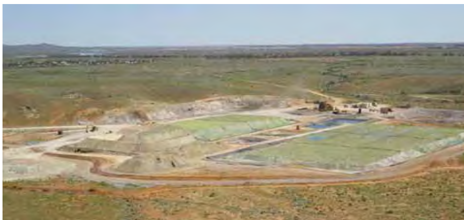
Leigh Creek Copper leach pad and processing facilities
