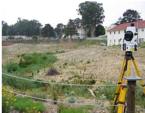
At Site 2, looking upstream, nine months after construction, showing vegetation growth
