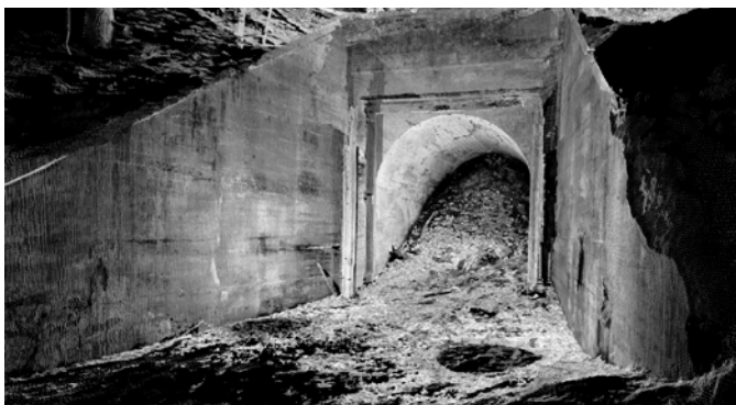
FARO S350 data of collapsed Wrays Hill tunnel exit
