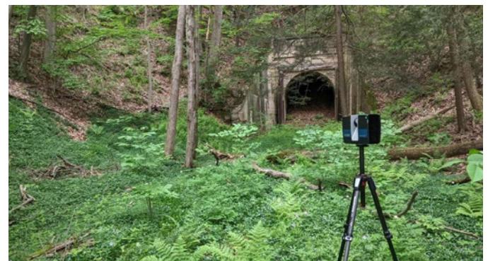
FARO S350 scanner in front of Wrays Hill tunnel exit – note the surrounding vegetation and condition of the outside rail lines
