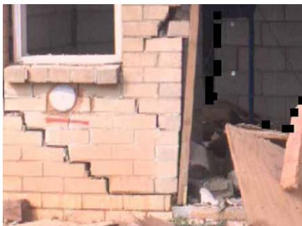
Damage to the house in terms of its overall stability, as well as the destruction of individual materials, can be clearly seen on images acquired and registered automatically to the 3D data by the I-Site 4400
