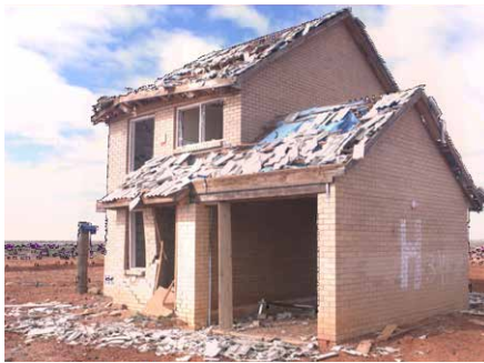
Damage to the house
