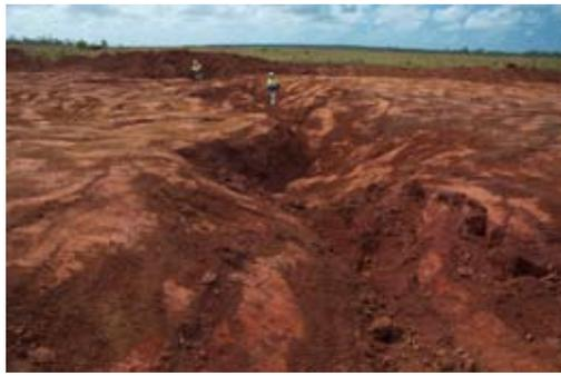
Overburden removal uncovered hidden anomalies, such as an old drainage line
