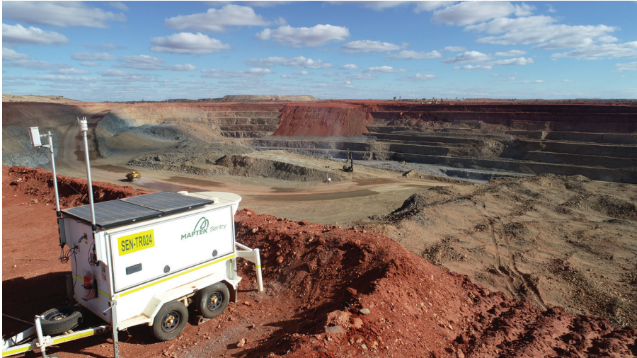
Sentry trailer set up to monitor pit wall
