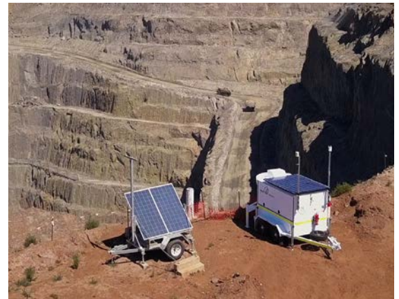
Sentry set up to monitor the western wall of the Giant Pit
