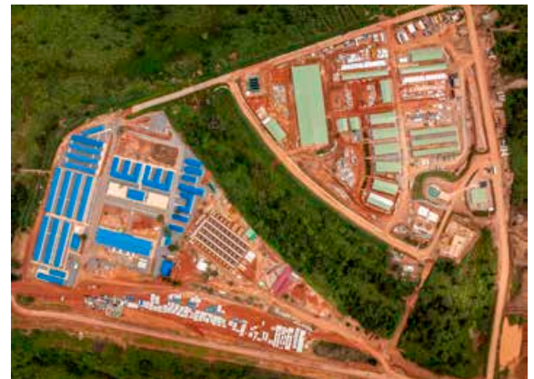
View of Rio Tinto's Simandou project in Guinea, West Africa
